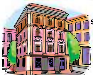
multistoreyed block of flats
